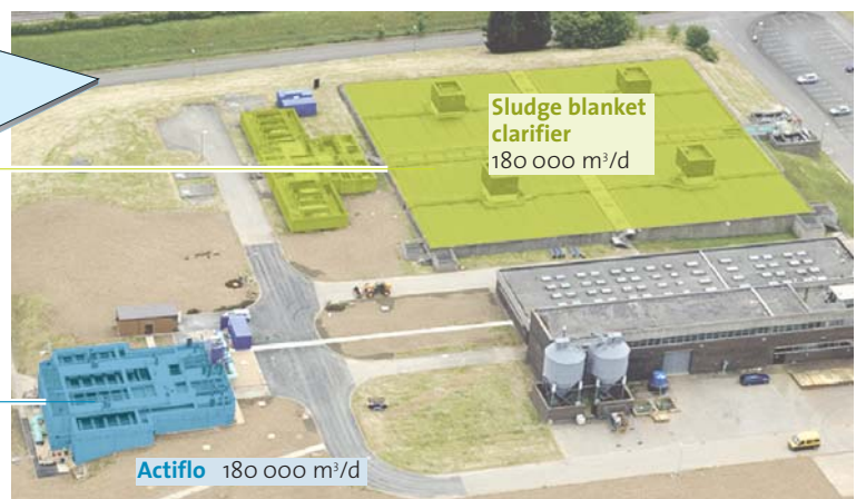
Overview of the Iver plant, London - Heathrow (United Kingdom). Clarification, interozonation and granular activated carbon filtration for drinking water production.
